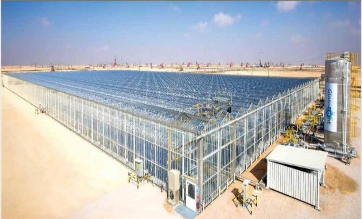
**Fuente:** GLASSPOINT SOLAR, INC. First enclosed-trough solar steam generation pilot for EOR applications.
