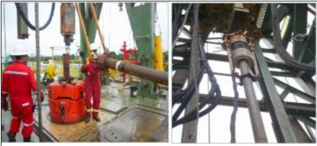
Figura 22. Casing Drive System (CDS)
