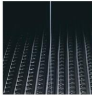
Scan test showing leak indicated by a smoke trail.
