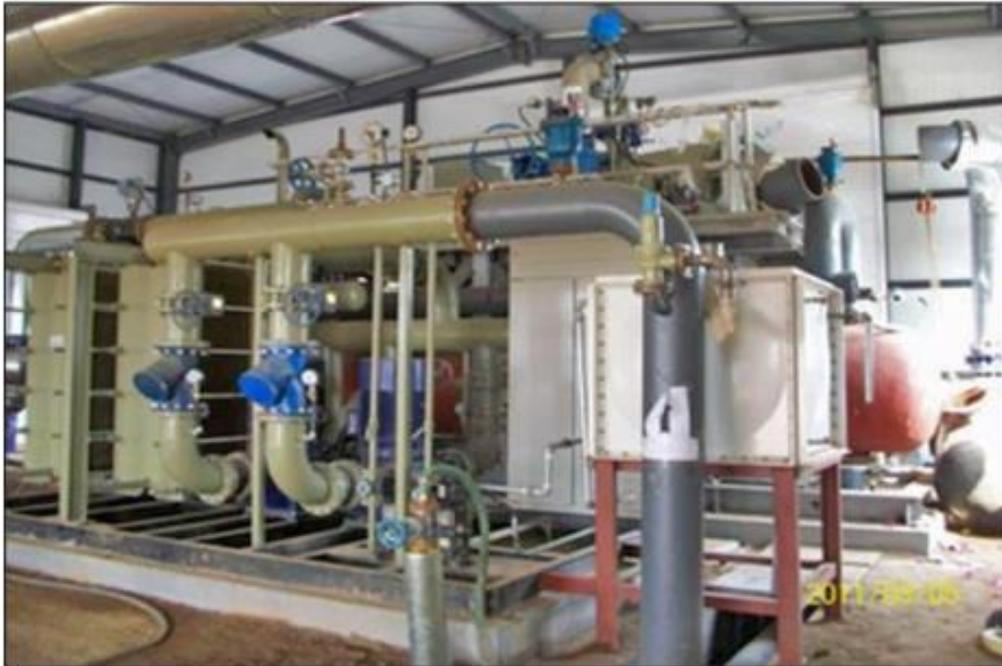
Nota: Tomado de: Xin, S., Liang, H., Hu, B., & Li, K. (2012). A 400 kW geothermal power generator using co-produced fluids from Huabei oilfield. Transactions - Geothermal Resources Council, 36 1, 219–223.
